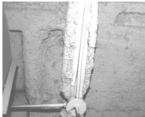
Many buildings have asbestos sprayed onto beams and decks as fireproofing.
